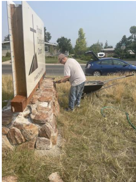
Pastor Charles fixing the stone work at the base of our sign.
